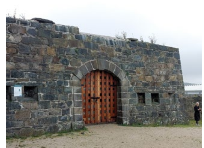
3.3.9 Original Entrance with Modern Gates, West Side (Insall, 2021)
