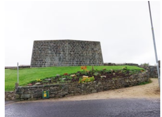
3.3.15 The Blockhouse, View from the Road (Insall, 2021)
