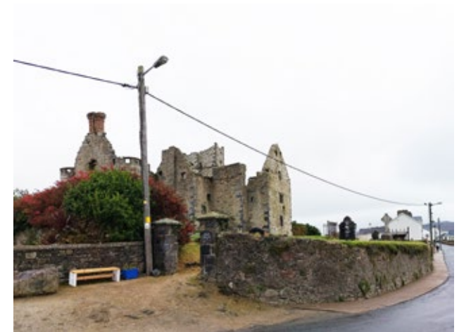
3.5.54 Wall Surrounding Site (Insall, 2021)
