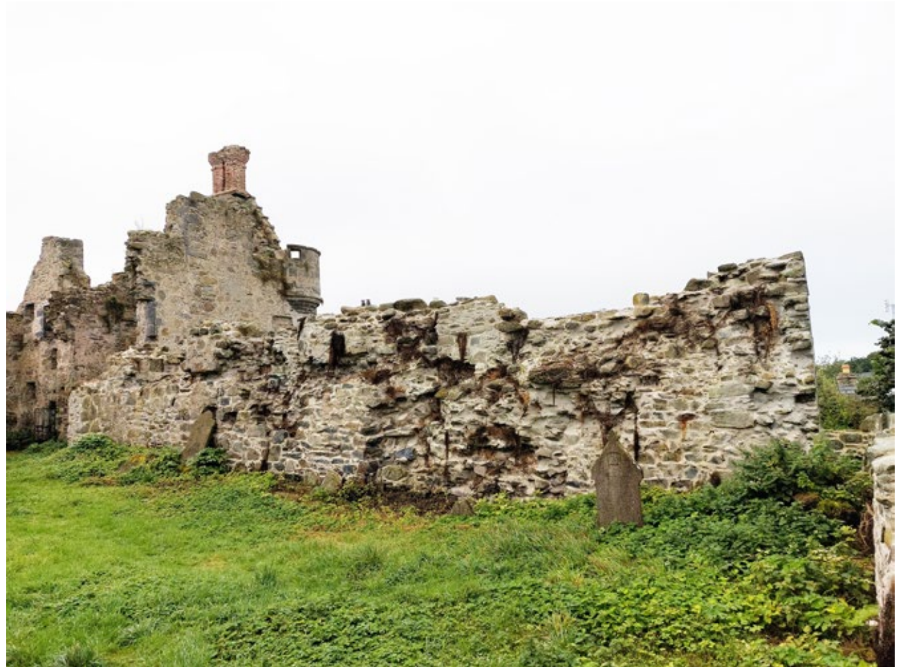
3.5.50 Internal View of West Elevation of Domestic Range Area (Insall, 2021)
