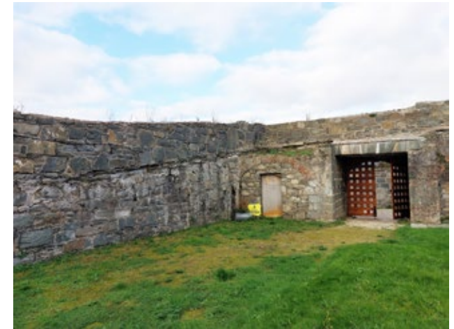
3.3.7 Original Guard House and Entrance with Modern Gates (Insall, 2021)
