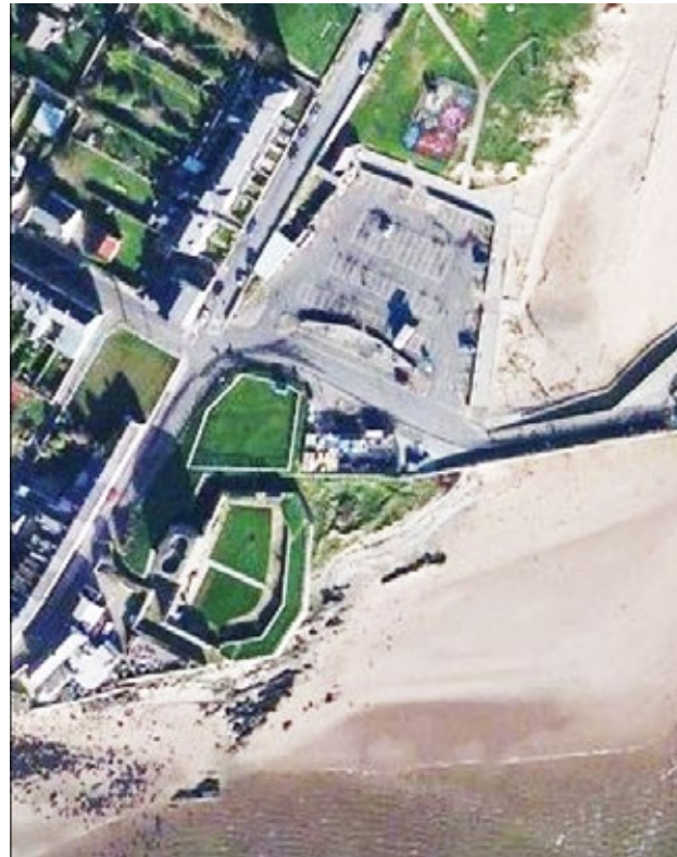
3.2.1 Aerial View of the Battery Fort (MacGabhann Architects)
