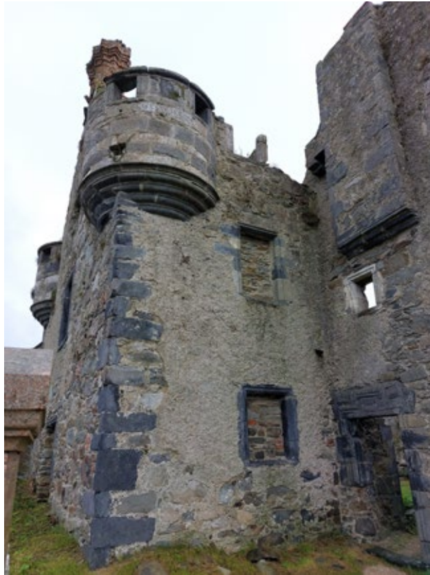
3.5.24 South Elevation of Nave (Insall, 2021)
