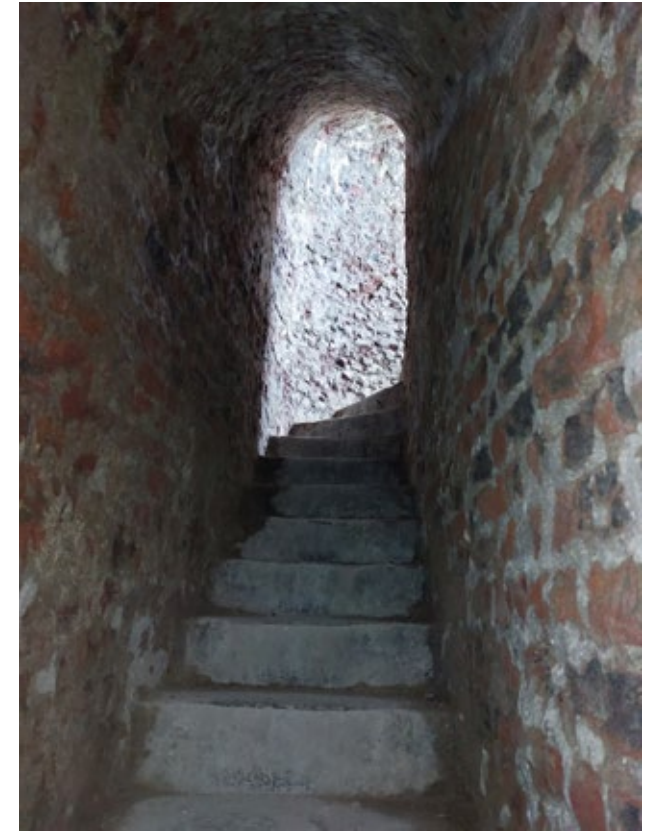
3.3.22 Staircase Connecting First Floor and Roof (Insall, 2021)
