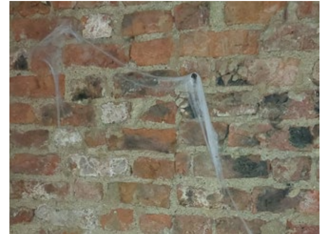
3.3.19 Showing Infilled Ventilation Opening (Insall, 2021)
