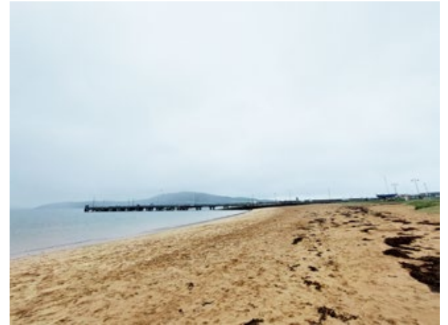
3.1.3 Pier with 20 th -century Extension (Insall, 2021)
