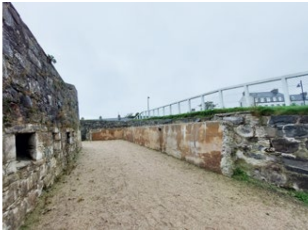
3.3.25 Remnant of WWI Water Tank in Northwest Corner of Ditch (Insall, 2021)
