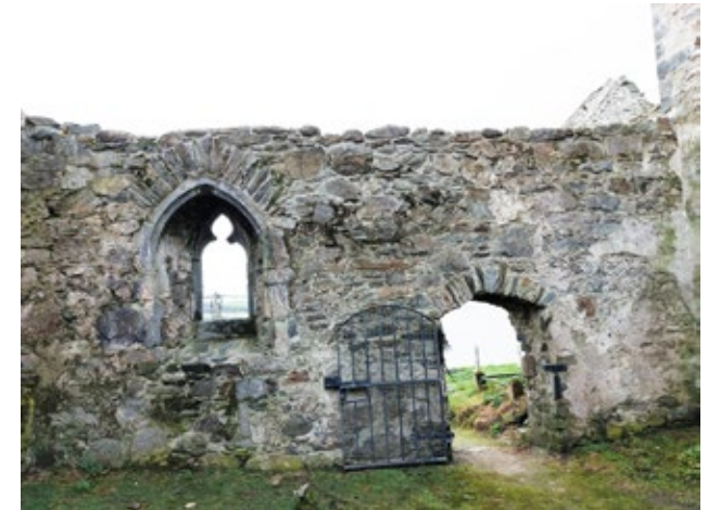
3.5.6 Internal View of South Elevation of Chancel (Insall, 2021)
