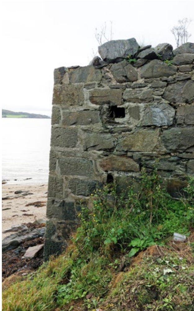
3.3.27 Openings in Retaining Wall, End of South Ditch (Insall, 2021)
