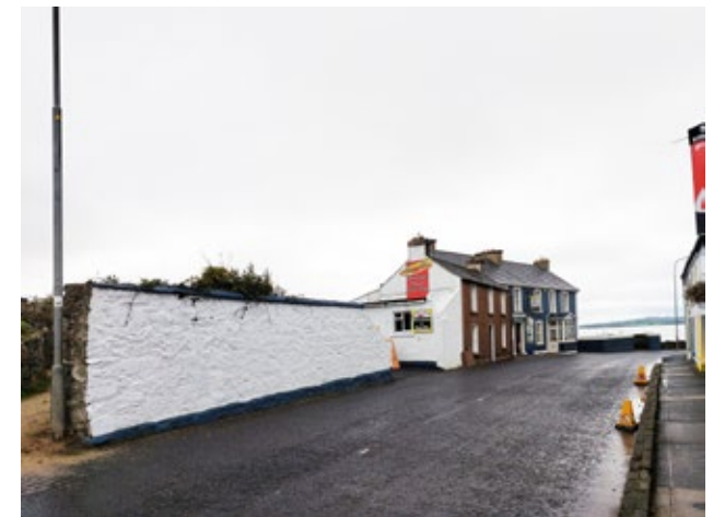
3.3.31 Buildings on Former South Grass Glacis (Insall, 2021)
