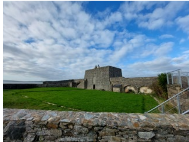
3.3.1 The Battery Fort Courtyard (Insall, 2021)
