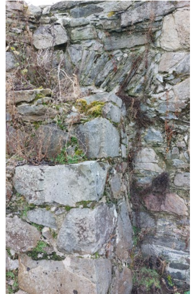
3.5.11 Visible Arch of Blocked Doorway, North Elevation of Chancel (Insall, 2021)
