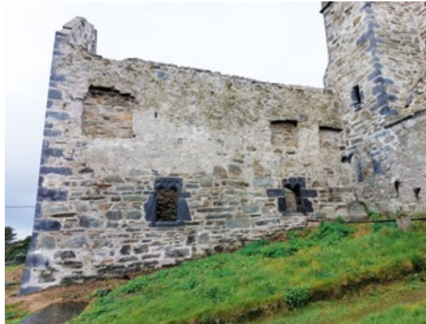
3.5.39 East Elevation of Transept (Insall, 2021)
