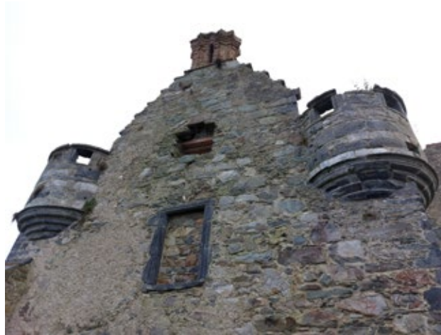
3.5.22 Gable of West Elevation of Nave (Insall, 2021)
