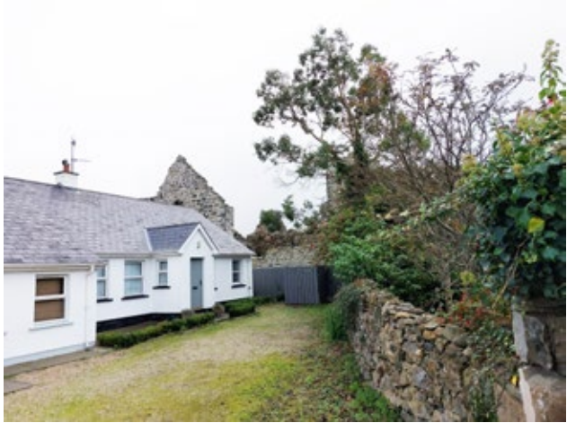
3.5.47 Partial View of North Elevation of Domestic Range (Insall, 2021)
