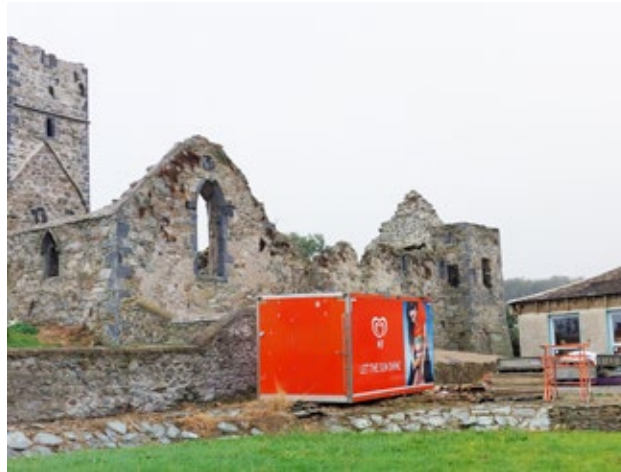
3.5.43 East Elevation of Domestic Range, with Chancel to the South (Insall, 2021)
