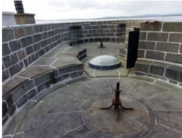
3.3.16 The Blockhouse Roof (Insall, 2021)
