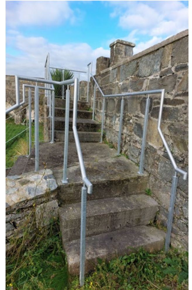
3.3.11 Northern Access to East (Coast) Embankment (Insall, 2021)
