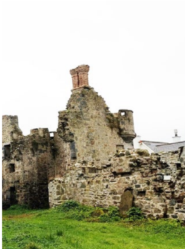
3.5.26 Partial View of North Elevation of Nave (Insall, 2021)
