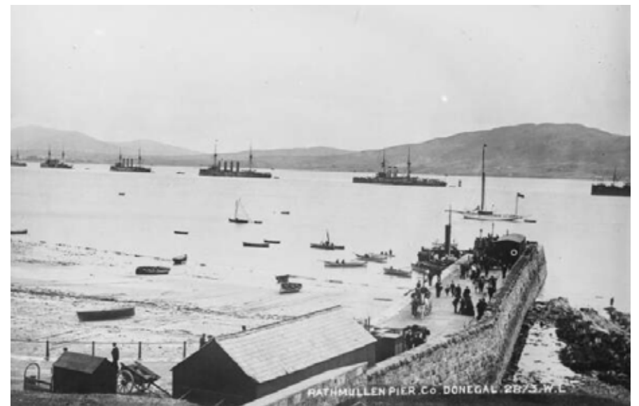
2.1.9 Photograph of Rathmullan Pier c. 1870-90 (Eblana Photograph Collection, NLI - EB_2873)
