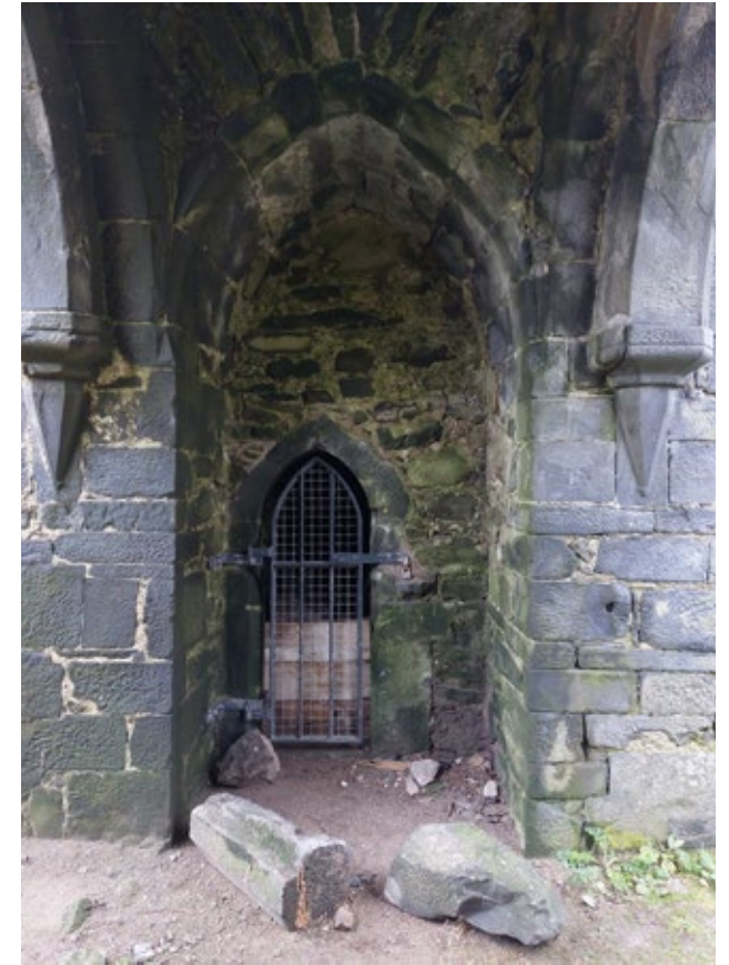
3.5.18 Entrance to Spiral Staircase of Tower (Insall, 2021)
