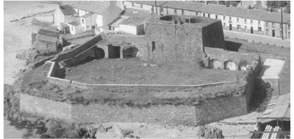
2.3.11 Aerial photograph showing the battery fort from the mid-20 th century showing the guns and magazines in the courtyard removed
