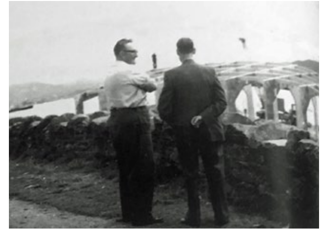
2.1.11 Photograph of the potato store during construction, 1960
