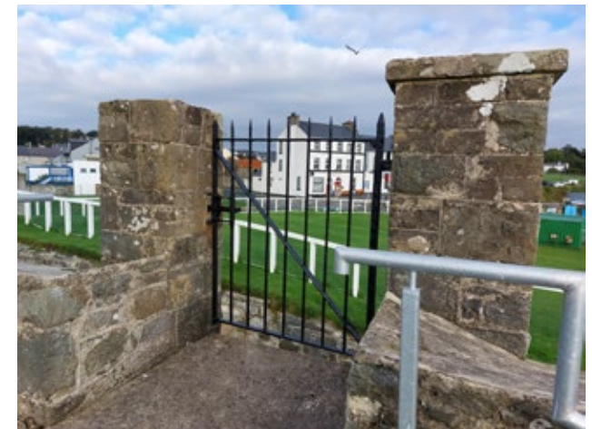
3.3.3 WWI Stone Piers and Gate (Insall, 2021)
