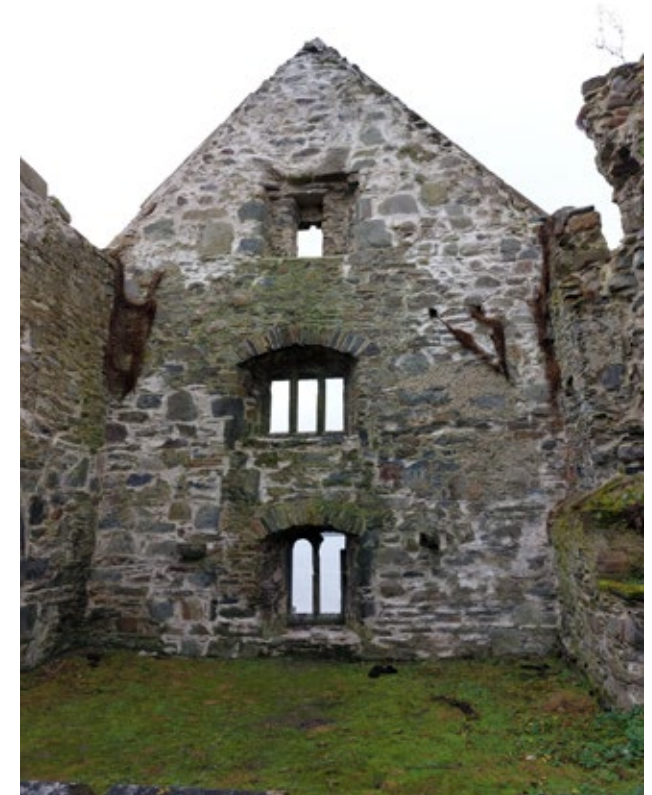
3.5.37 Internal View of South Elevation of Transept (Insall, 2021)
