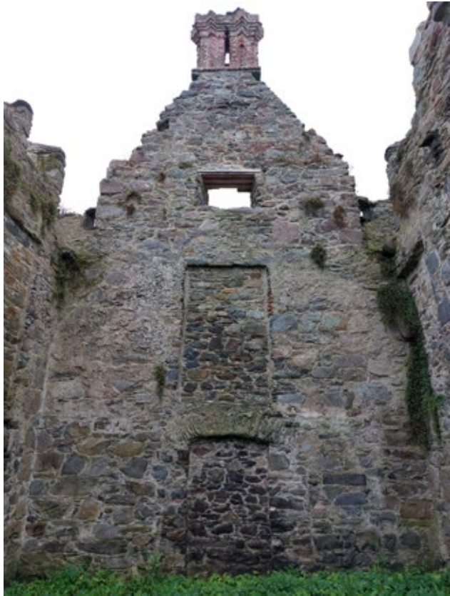
3.5.23 Internal View of West Elevation of Nave (Insall, 2021)
