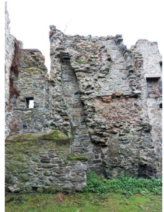
3.5.35 Internal View of West Elevation of Transept (Insall, 2021)
