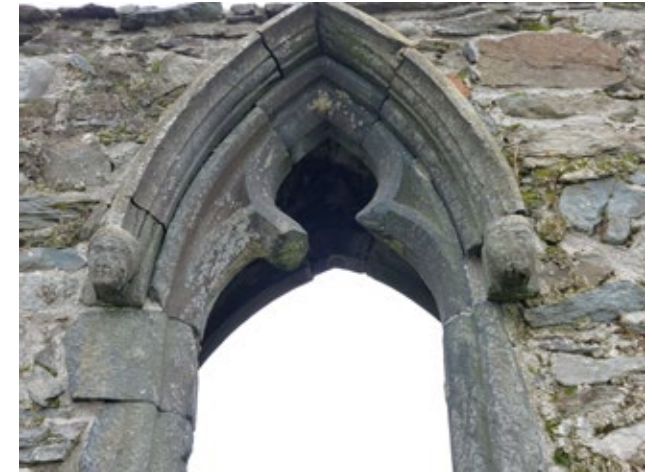
3.5.5 Detail of Window, South Elevation of Chancel (Insall, 2021)
