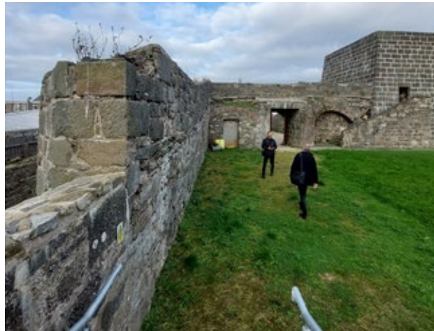
3.3.6 Southwest Corner of Courtyard, showing Entrance and Guard Room (Insall, 2021)
