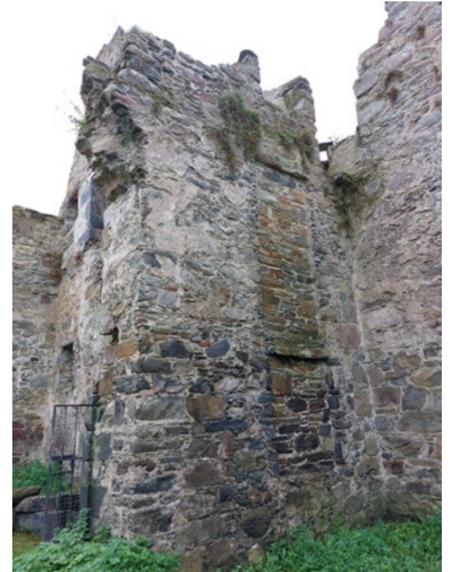
3.5.25 Internal View of South Elevation of Nave (Insall, 2021)
