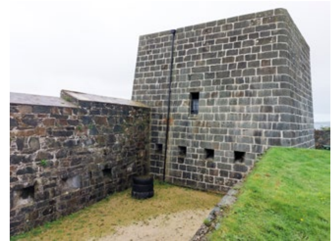
3.3.14 The Blockhouse, North View from the Ditch (Insall, 2021)
