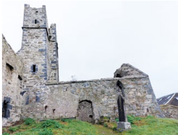
3.5.4 South Elevation of Chancel and Tower (Insall, 2021)
