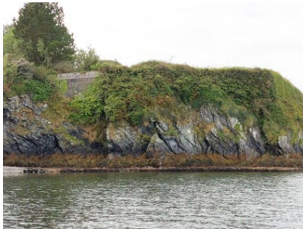
3.1.11 Battery on Inch Island (Insall, 2021)
