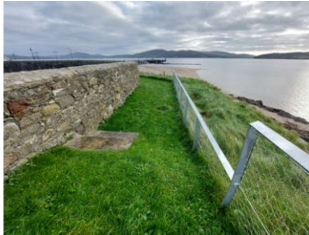
3.3.10 Lowering and Levelling of East (Coast) Embankment (Insall, 2021)
