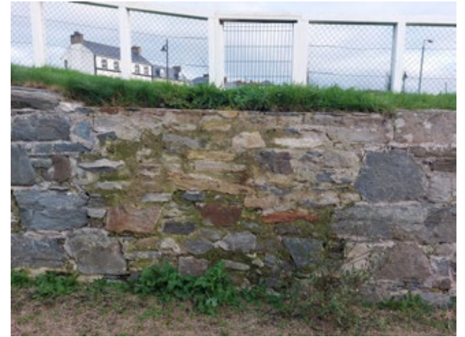
3.3.26 Rebuilt Section of Wall, North of Ditch (Insall, 2021)
