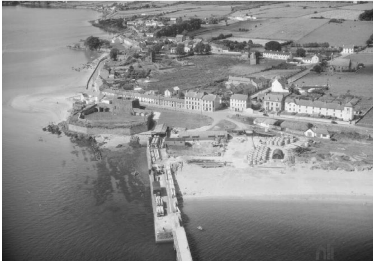
2.1.10 Photograph of Rathmullan showing Pier and Fort, 1954 (Morgan Aerial Photograph Collection, NLI - NPA MOR276)
