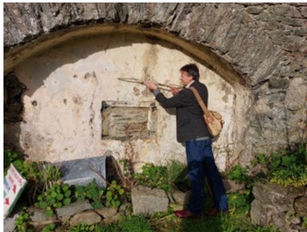
3.3.5 Showing the raised courtyard level resulting in a gunner being positioned too high for gun loops (Insall, 2021)
