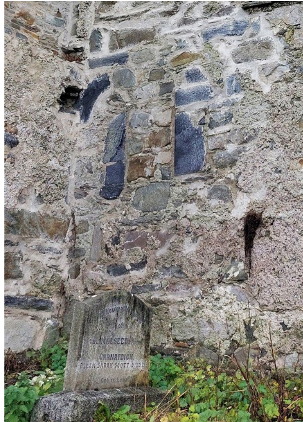
3.5.17 Ground Floor of South Elevation of Tower (Insall, 2021)
