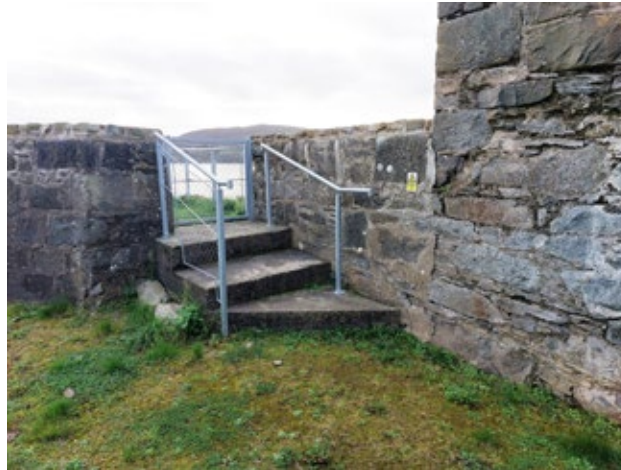
3.3.12 Southern Access to East (Coast) Embankment (Insall, 2021)
