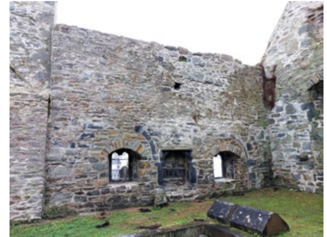
3.5.40 Internal View of East Elevation of Transept (Insall, 2021)
